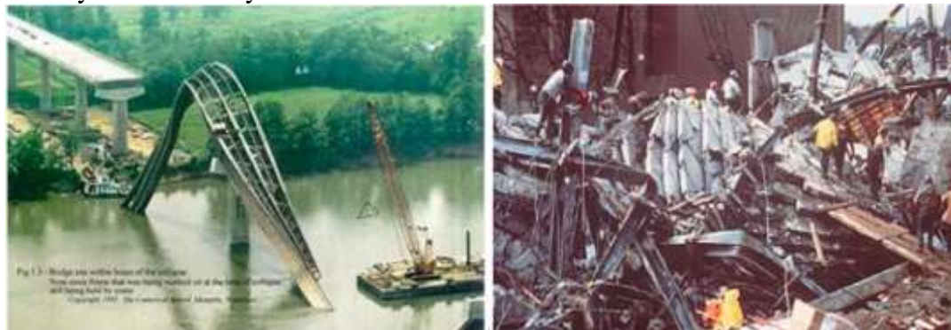
Fig.7:- Collapse of Tennessee Highway 69 bridge and Bridgeport Connecticut (US) steel frame (Source: Derseh et al., 2023)
