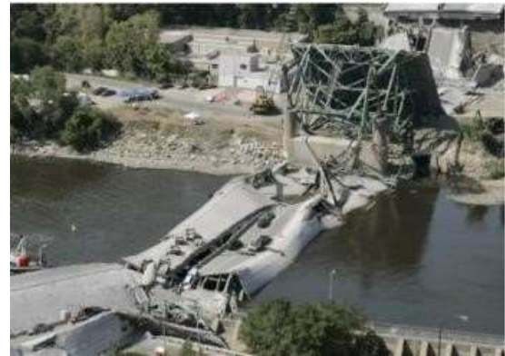
Fig.1:-I-35W steel deck truss bridge before and after the collapse (Source: Derseh et al., 2023)
