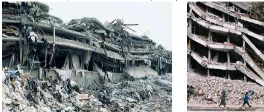
Fig.4:- Pancake collapse at Mexico and Turkey (Source: Derseh et al., 2023)
