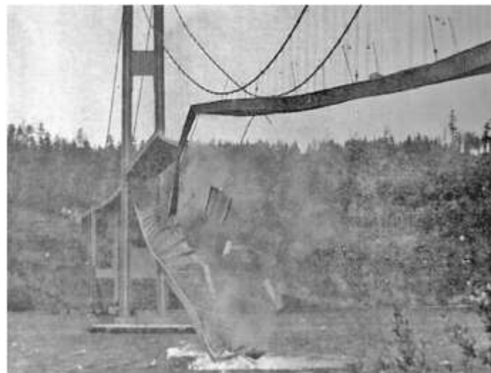
Fig.5:- Zipper-type collapse on Tacoma Narrows Bridge (Source: Derseh et al., 2023)
